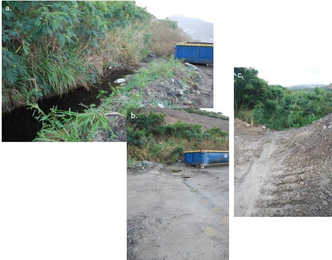
Figure 7. (a) Surface water ditch sampled along the road directly adjacent to the landfill. (b) A trench across the road drained the surface water ditch in (a) into the upland of the mangrove fringe pictured in (c). (c) Upland vegetation leading into the study region (mangrove fringe below). All pictures taken January 9, 2014 by K. Wilson.
